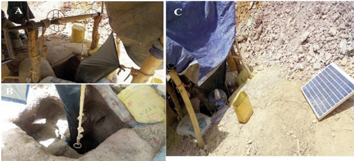
Illustration 1: hole dug by diggers (photo A), rope used by diggers to get down and raise up from hole (photo B) and holes ventilation system (photos C).
